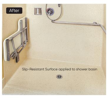
The showers were refinished to like-new condition including the application of Miracle Method's durable Slip Resistant Surface (SRS).
