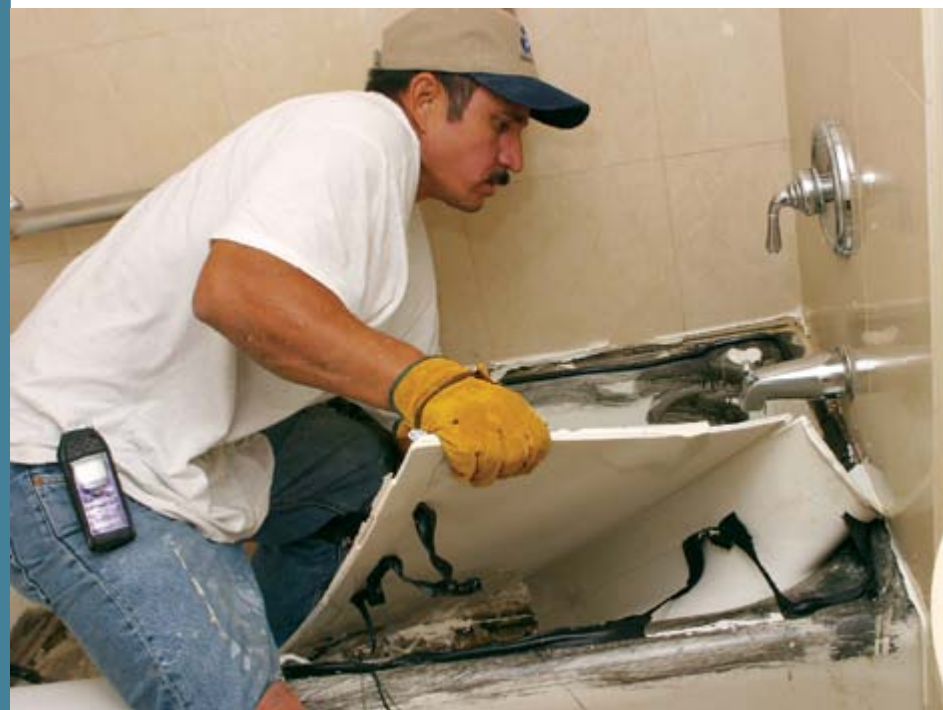
A Miracle Method technician removing a leaking tub liner.
